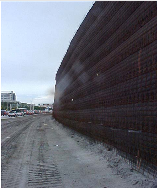
TEMPORARY WELDED WIRE WALL MAINTENANCE OF TRAFFIC - PGA BLVD PALM BEACH, FL
