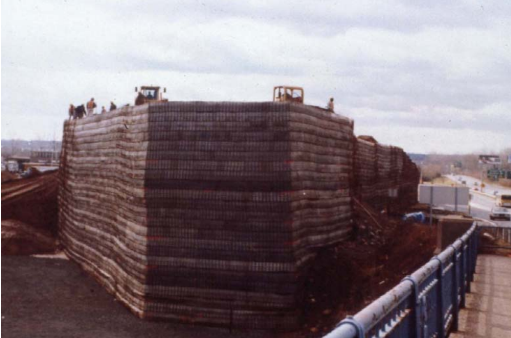
TEMPORARY WELDED WIRE WALL SURCHARGE WALL - CONNECTICUT
