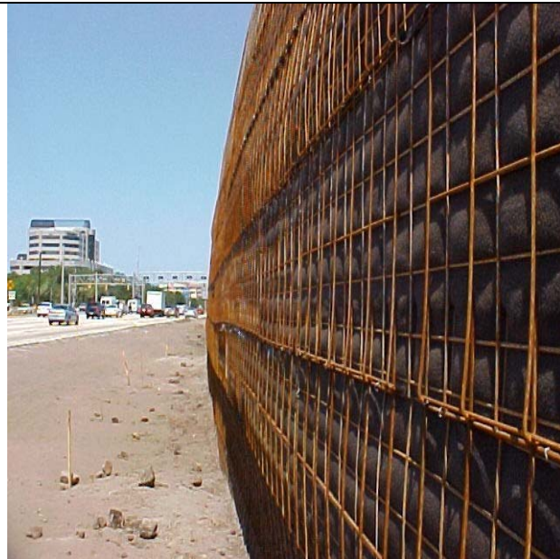
TEMPORARY WELDED WIRE WALL MAINTENANCE OF TRAFFIC - PGA BLVD PALM BEACH, FL
